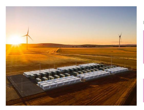
This is the Tesla battery at Hornsdale in Australia. It can store 129 MWh, a settlement of 2,000 houses would have the same storage capacity. It can deliver or store 100 MW, a settlement of 3,000 houses would have the same capacity.
